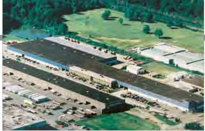
South Plainfield, NJ
